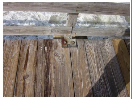
**Description:** View over Pier #20. As the pier begins to go over water seaward, the impact of the sea environment is increasingly harsh on wood and metal hardware. Note the sign of decay on the board immediately to the left of the post. Note a decaying board on the left.
