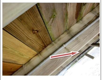
**Description:** Typical view of the substructure framing and the condition of the decking underside from Pier #18. Note proliferation of algae between the gaps. Note multiple replacement boards. Also note some loose cross-bracing hanging beyond.
