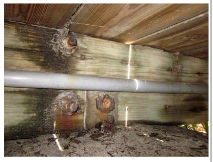
**Issue:** The rail post thru-bolt connectors and anchor bolt/ clip angle assembly on this side are undergoing severe corrosion as well.
