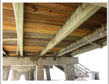
Description: General view of the decking underside and the substructure, looking seaward at Pier #5. Note the water piping and electrical conduits. Also note random horizontal cross-bracing. Note the accumulation of wet beach sand and debris falling from the foot traffic on either side of the stringer splice burying the anchor bolt/clip angle assembly causing accelerated corrosion of the metal hardware.
