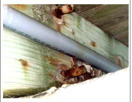
**Issue:** See preceding issue. Note hex-nuts and washers have corroded away and cleared from the end of the rail post thru-bolts causing potential faulty structural connections.
