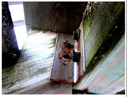
**Issue:** Stair stringer/deck stringer vertical connection assembly display severe corrosion of the metal hardware.
