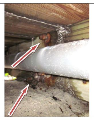
**Issue:** Electrical conduits and small water pipes are strapped to the stringers with plastic straps or in some cases plastic hangers. Note the corroding washers and complete loss of hex-nuts, of both of the thru-bolt connectors, to corrosion, at the base of a rail post over Pier #3. The anchor bolt and clip angle appear to have completely corroded away as well.
