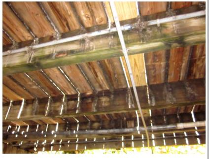
**Description:** View of the decking underside in between Pier# 2 and Pier #3. The underside surface and the stringers appear to be in satisfactory condition. Note water piping and electrical conduits strapped to the stringers.
