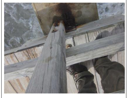
**Issue:** The connection assembly on the pier is the most vulnerable to sea spray that brings split and decay on wood, and promotes accelerated corrosion of metal hardware.
