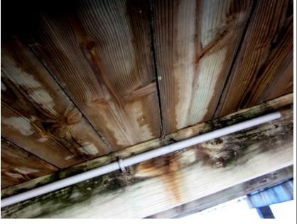
In stormy day and high waves the deck is being washed in sea spray for the duration. Note the boards are soggy from such weather event. Note the small pipe/conduit appears to have been broken off.
