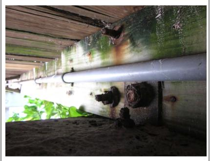
**Issue:** The rail post thru-bolt connectors and anchor bolt/ clip angle assembly on this side are undergoing severe corrosion as well. Note the top thru-bolt washer and hex-nut have been corroded away.
