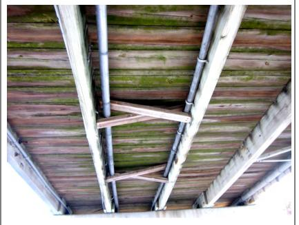
**Description:** Typical view of the substructure framing and the condition of the decking underside in the vicinity of Pier #11.
