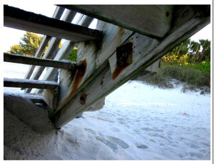
**ISSUE:** Almost all of the stair assembly thrubolt connections display severe corrosion of the metal hardware.
