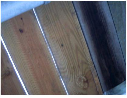
**Description:** Typical view of the substructure framing and the condition of the decking in the vicinity of Pier #12. Note the multiple replacement boards besides the old boards.
