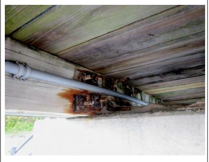
**Issue:** View of the same assembly on the inside face, which reveals severe corrosion of almost all the thru-bolts.
