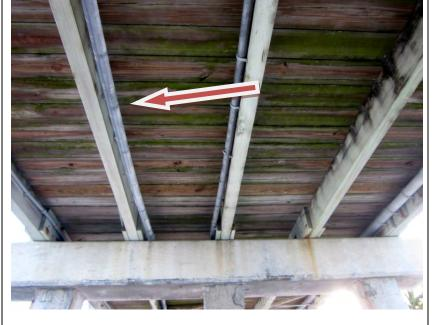
**Issue:** The stress caused by the movement of the main power supply conduit is beyond the working strength of these thin plastic pipe straps. Note the conduit has dropped away from its strapping alongside the stringer.
