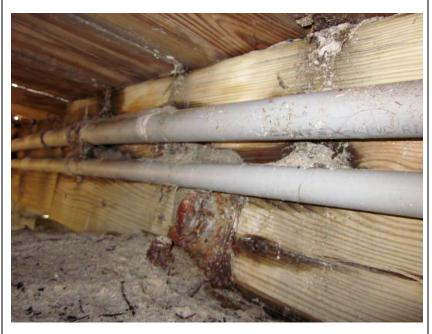
**Issue:** View of an inside stringer anchor bolt/clip angle assembly which is normally buried under the beach sand causing accelerated corrosion of the metal hardware.
