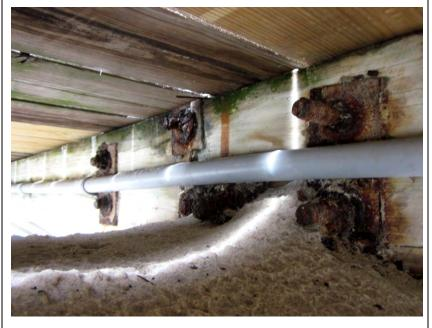
**Issue:** View of the same assembly on the interior face, which reveals severe corrosion of almost all the thru-bolts.
