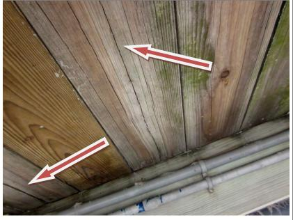
**Description:** Typical view of the substructure framing and the condition of the decking underside from Pier #10. Note boards with split fiber.
