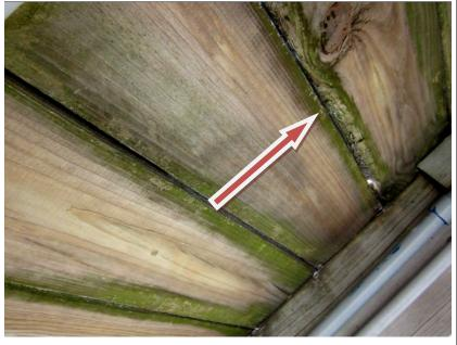
**Description:** Typical view of the substructure framing and the condition of the decking underside from Pier #17. Note proliferation of algae between the gaps. The board on the right is beginning to decay from the edge.
