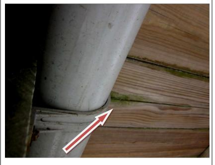
**Description:** Typical view of the substructure framing and the condition of the decking underside from Pier #16. Note the fiber split in the middle board despite it fresh appearance. The start of algae growth within the split indicates that moisture is migrating through the split from top to bottom. This is where wood decay is naturally takes root.
