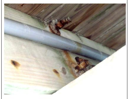
**Issue:** Pier #9. See preceding issue. Note the two hex-nuts and a washer have corroded away and cleared from the end of the rail post thru-bolts causing potential faulty structural connections.
