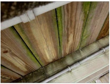
**Description:** Typical view of the substructure framing and the condition of the decking underside from Pier #7. Note algae growth between boards.
