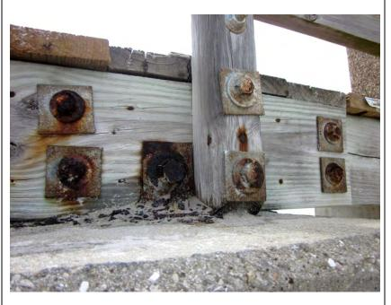
**Description:** View on the exterior face of the splice assembly at Pier #5, where extra pairs of thru-bolt are used to stiffen up the outside stringer before the stair landing opening on the right.
