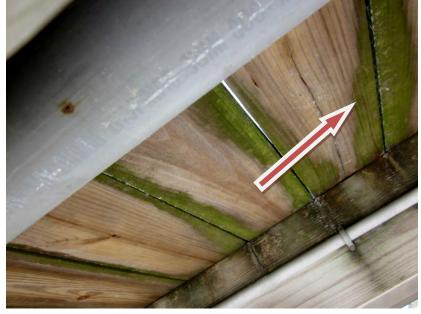
**Description:** Typical view of the substructure framing and the condition of the decking underside from Pier #16. Note proliferation of algae between the gaps.
