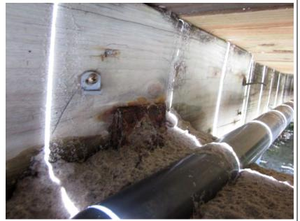
**Issue:** See preceding issue. Note the broken pipe straps leaving the conduit/pipe unsupported.
