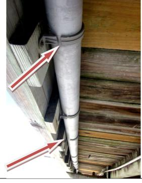
**Issue:** The stress caused by the movement of the main power supply conduit is beyond the working strength of these thin plastic pipe straps.
