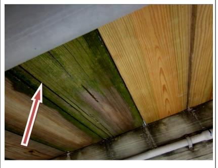
**Description:** Typical view of the substructure framing and the condition of the decking underside from Pier #7. Note a board with split fiber and covered with algae which accelerates wood decay. Note replacement board.
