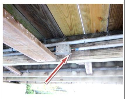
**Issue:** The movement of the deck under wind gust can pull pipe/conduit out of its joint and/or rip a pipe segment out of its strapping.
