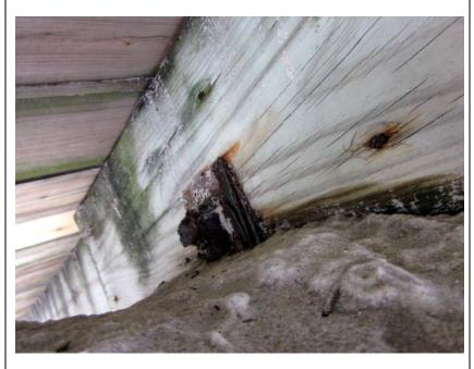
**Issue:** View of repeated pattern of severe corrosion of thru-bolt and anchor bolt assembly due to near-constant wetness condition on top of the pile cap and the lack of direct sunlight and airflow to help accelerate drying of all components under the decking.
