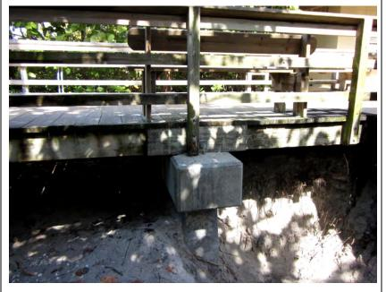
**Description:** View of the rectangular precast concrete bent and the deck and railing at Pier #2. Pier #1 is to the right immediately behind the Male Restroom rear wall.
