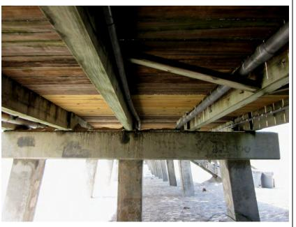
**Description:** General view of the decking underside and the substructure, looking seaward at Pier #4. Note the water piping and electrical conduits. Also note random horizontal cross-bracing.
